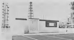
New Process Shelter near Alky Plant.
